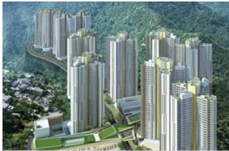
Public Rental Housing and Subsidized Sale Flats Development at Queen's Hill Site 1 BEAM Plus Neighbourhood Platinum Rating 2018
