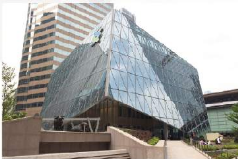
Exchange Square Forum Redevelopment 交易广场第三期
