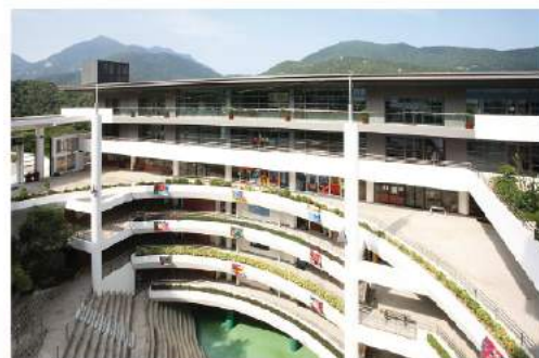
Hong Kong International School Expansion Tai Tam Campus 香港国际学校大潭校园
